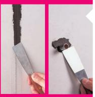
Joints should be reinforced with the supplied ARDEX Self Adhesive Mesh Scrim prior to applying MIX ONE. Apply MIX ONE with a spatula, pallet knife or trowel, sealing joints in corners and filling holes and gaps around pipes.
